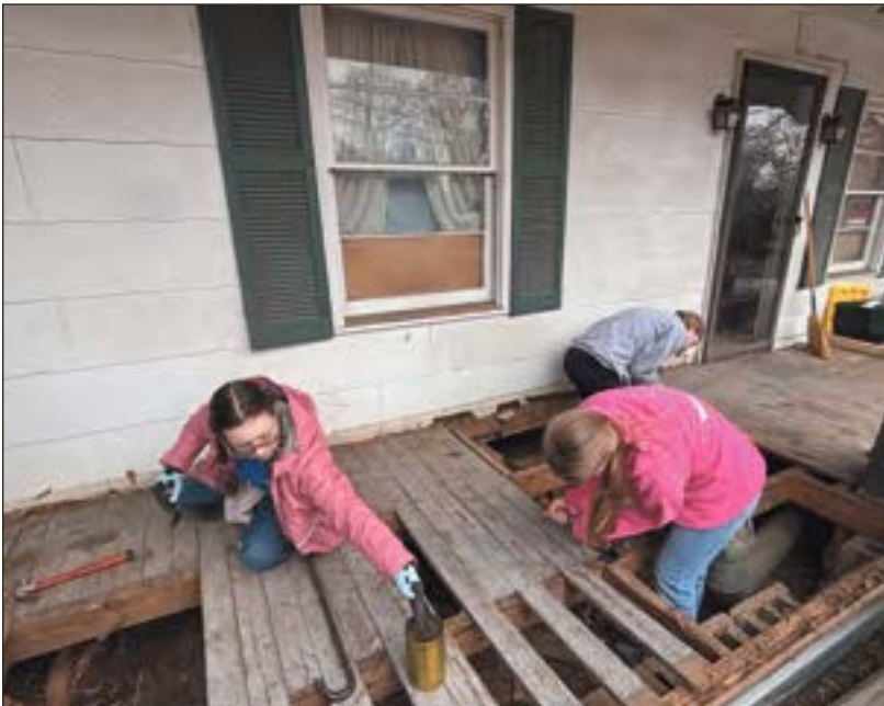
One of the homes needed porch repairs.
