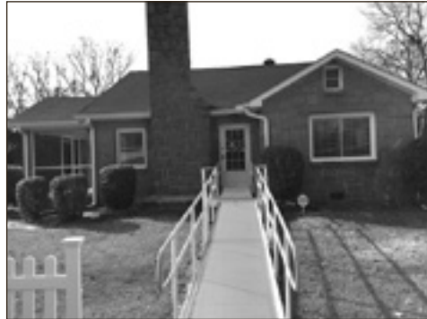
The Stone House is one of the few houses in Blythewood constructed with Winnsboro Blue Granite.
