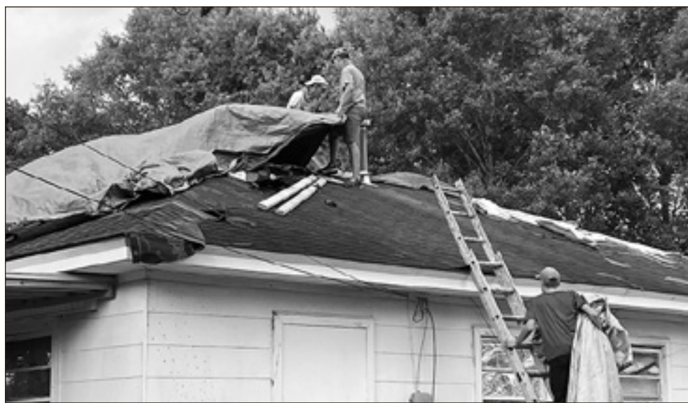
Roofwork was a big part of this home’s repairs.
