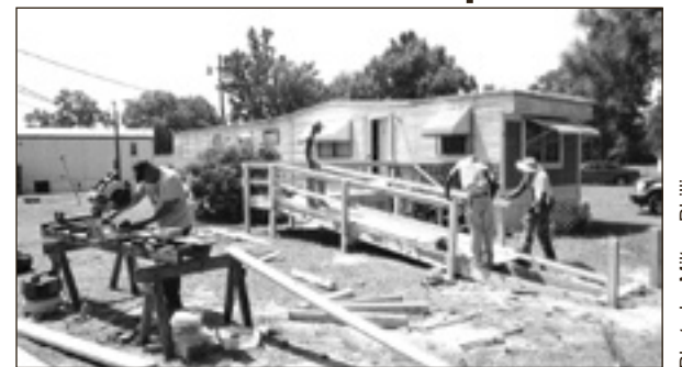
Men build ramps for people in need.
