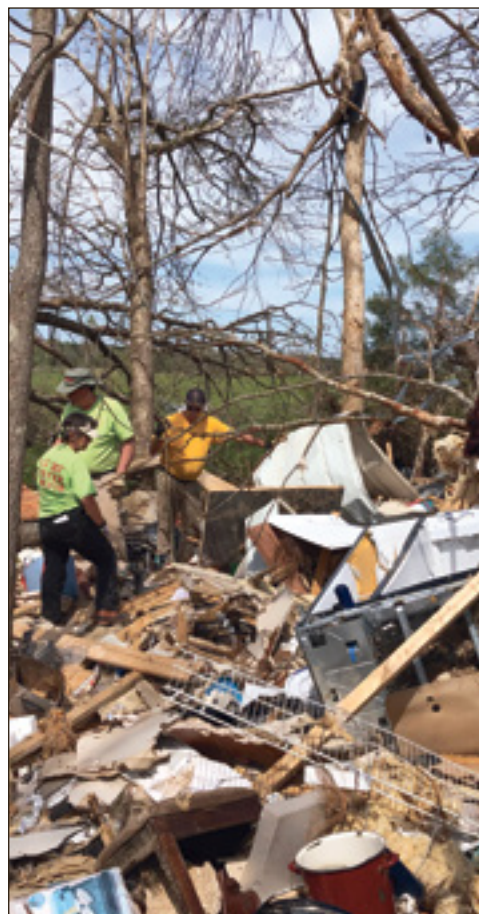
Team members picked through debris to help families find items to help them grieve.
